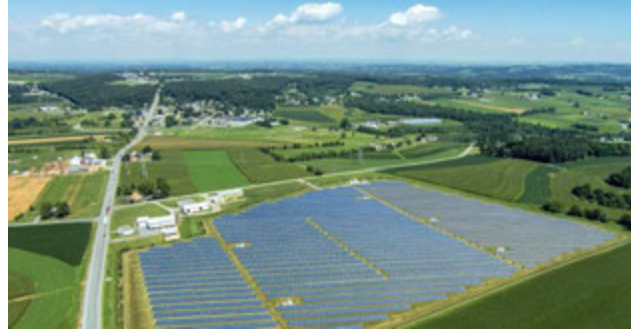
5 MW community-scale system
